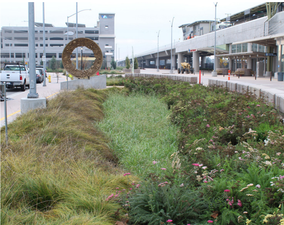
Berryessa Station Bioretention Basin
