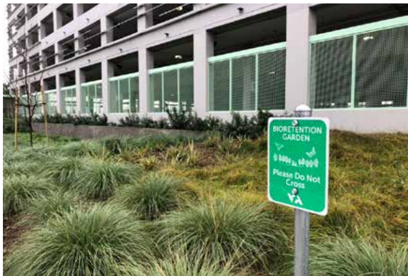
Figure 15: Bioretention Basin with Safety Signage
