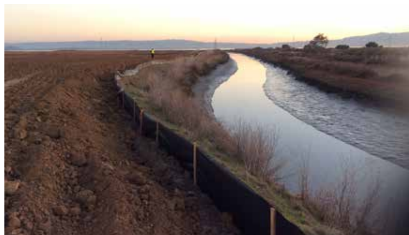
Figure 5: Temporary Perimeter Sediment Control with silt fence
