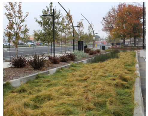
Milpitas Station Bioswale
