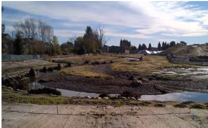
Figure 4: Final site erosion controls with jute blankets and hydroseed.
