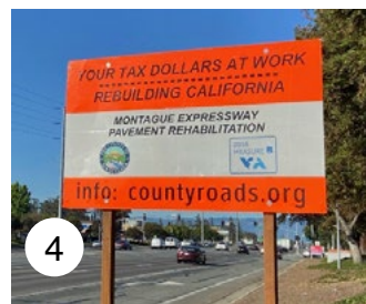
Pavement rehabilitation construction notice signage
