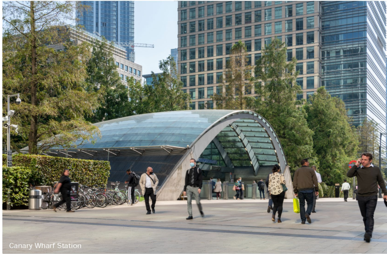
Canary Wharf Station
