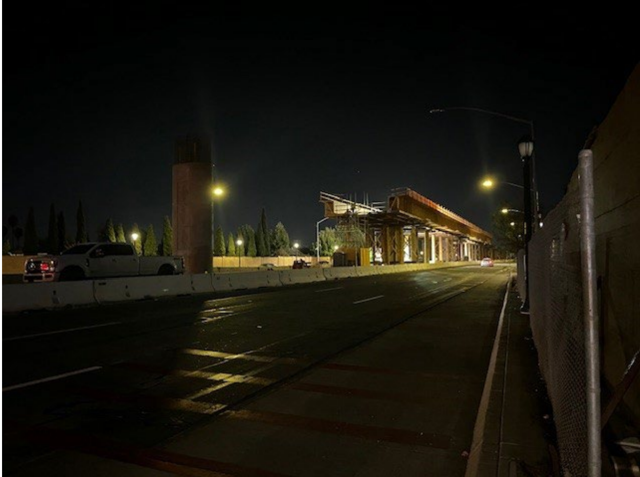
View of Southbound Capitol Expressway, Friday, November 15, 2024. Construction crews worked on the wooden structure that will support the bridge while it is being built (falsework), located in the median of Capitol Expressway between Ocala Avenue and Story Road. [Photo by VTA/EBRC LFP].
