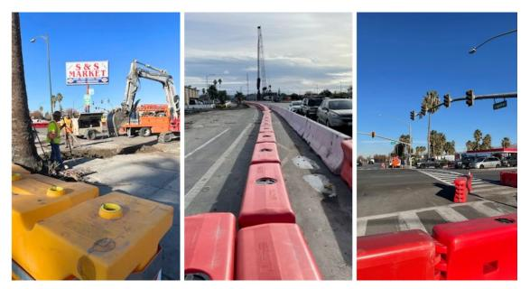
(Left to Right) – Foundation work for the elevator tower for the aerial VTA Story Road Station, close to Chevron and S&S Market. Pedestrian and bike pathways are clearly delineated throughout the construction zone. S&S Market is open during construction. [Photos VS/LFP].
