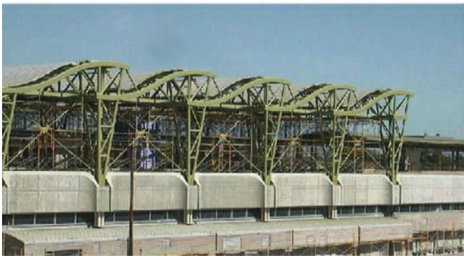
Elevated trackway at VTA's Berryessa/San Jose BART Station
