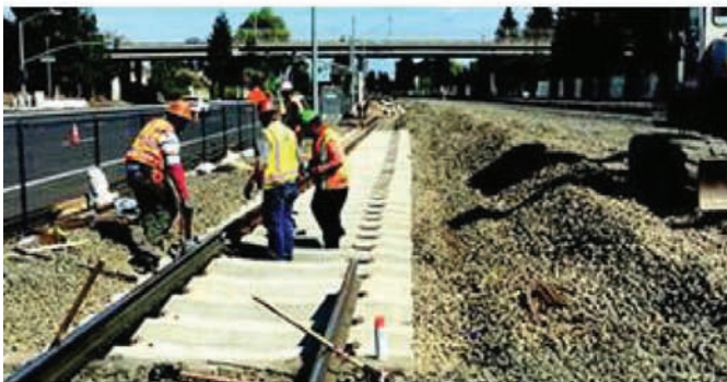
Award Winning Mountain View Double Track Project
