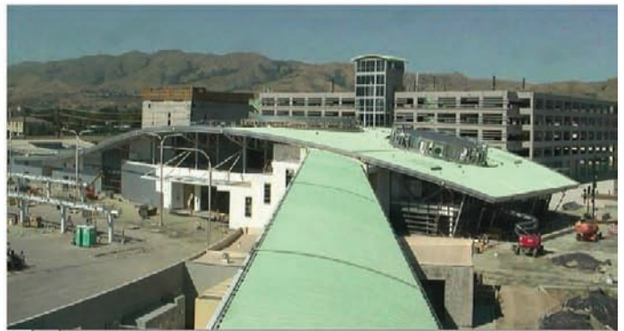
Pedestrian Overcrossing leading to VTA's Milpitas BART Station
