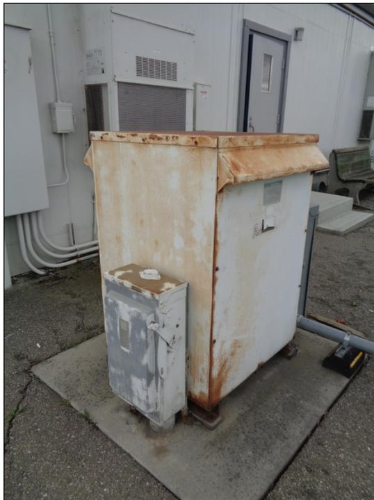
Photograph 12. Transformer for Building A.
